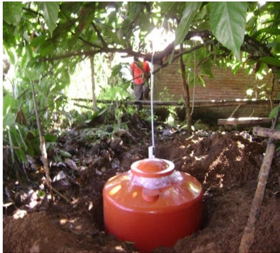
Gambar 10. Reaktor bahan fiber glass
