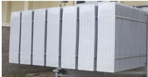
**Gambar 2.10** Pendingin Transformator
