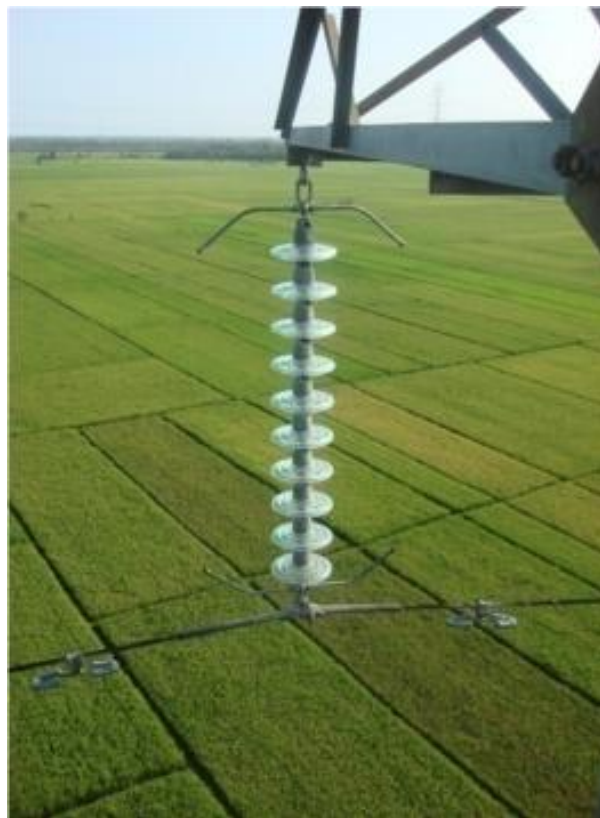
Gambar 2.8 Insulator single string
