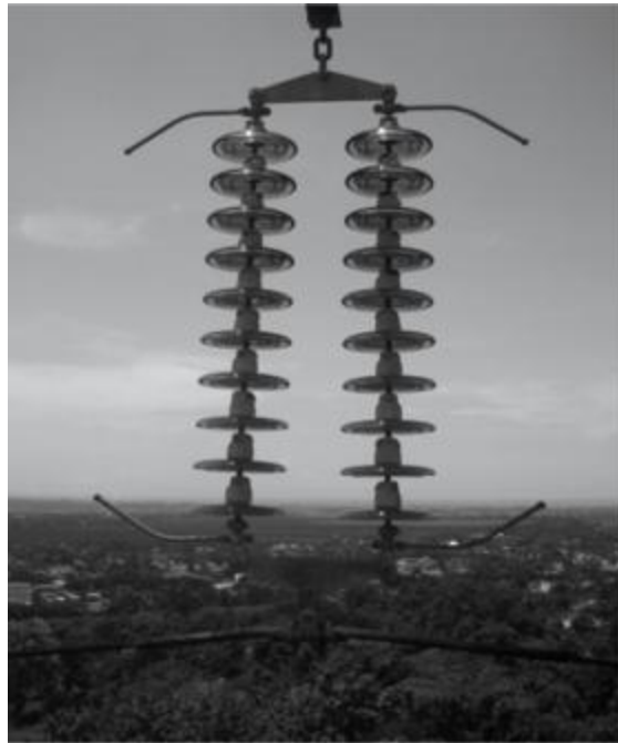
Gambar 2.9 Insulator double string
