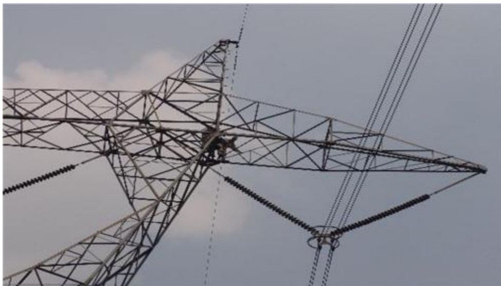
Gambar 2.6 Insulator "V" string
