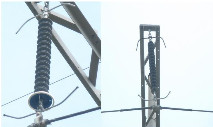
Gambar 2.4 Insulator long rod
