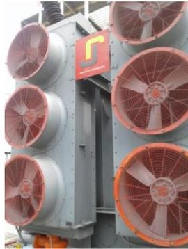
Gambar 2.12 Pendingin Transformator
