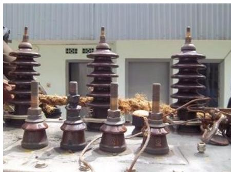
Gambar 2.10 Bushing Transformator
