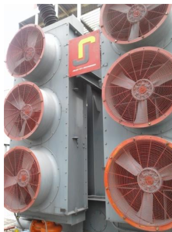
Gambar 2.11 Gambar Pendingin Transformator
