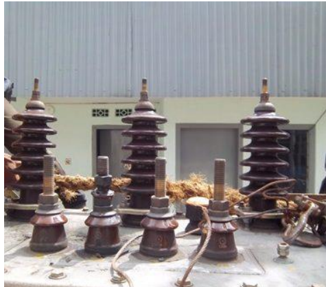
Gambar 2.9 Gambar Bushing Transformator
