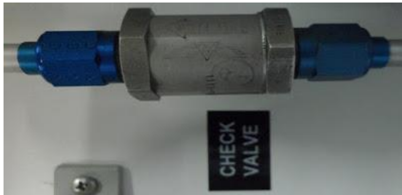
Gambar 2.3 Check Valve [7]
