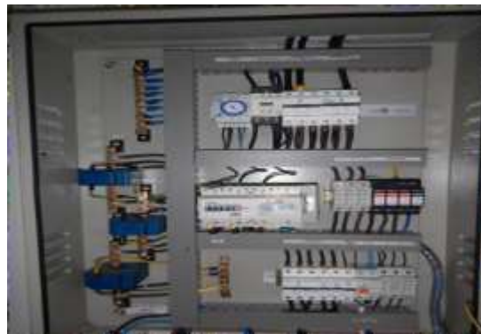
Gambar 2.21 Gambar Panel Distribusi AC
