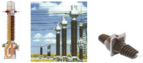
Gambar 2.12 Trafo Arus Pasangan Luar (Out-Door)
