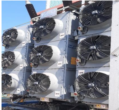
Gambar 2.11 Pendingin Transformator
