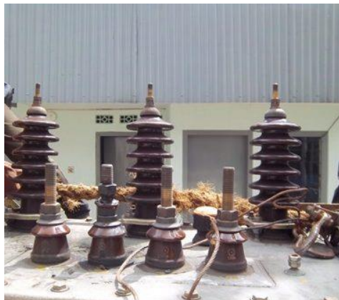
Gambar 2.9 Bushing Transformator
