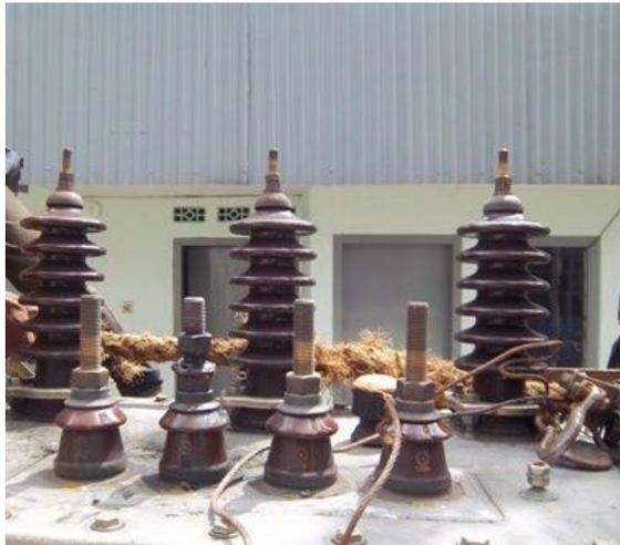
Gambar 2.7 Bushing Transformator
