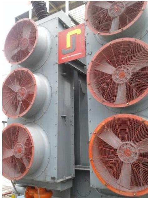
Gambar 2.9 Pendingin Transformator
