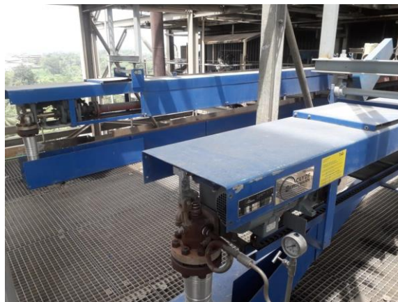
Gambar 2.12 Long retractable sootblower
