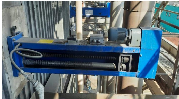
Gambar 2.14. Half Retractable Sootblower .
