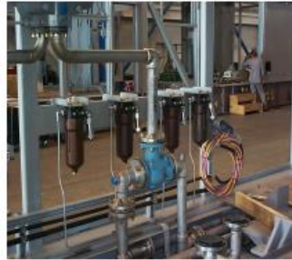
Gambar 2.25 Jacking Oil Pump Filters
