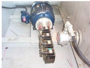
Gambar 2.24 Jacking Oil Pump
