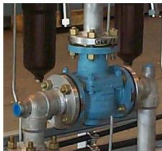
Gambar 2.20 Temperature Control Valve
