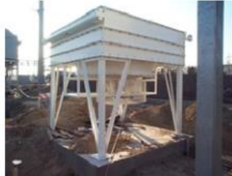
Gambar 2.19 Lube Oil Cooler
