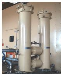
Gambar 2.21 Lube Oil Filters
