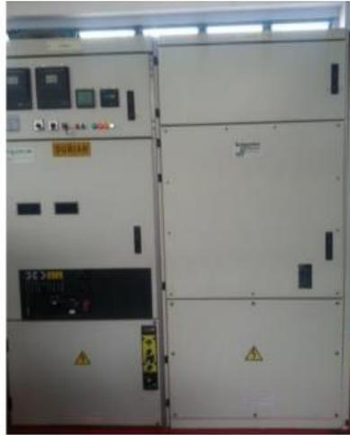
Gambar 2.8 Kubikel Bus Riser / Bus Tie (Interface) di GIS Kota Timur
