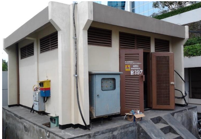
Gambar 2. 5 Gardu Beton
