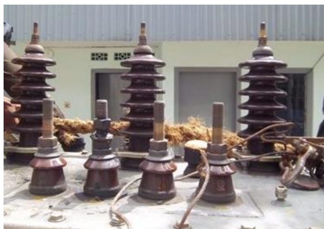
Gambar 2.7 Bushing Transformator
