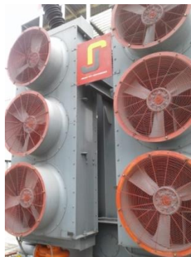
Gambar 2.9 Pendingin Transformator
