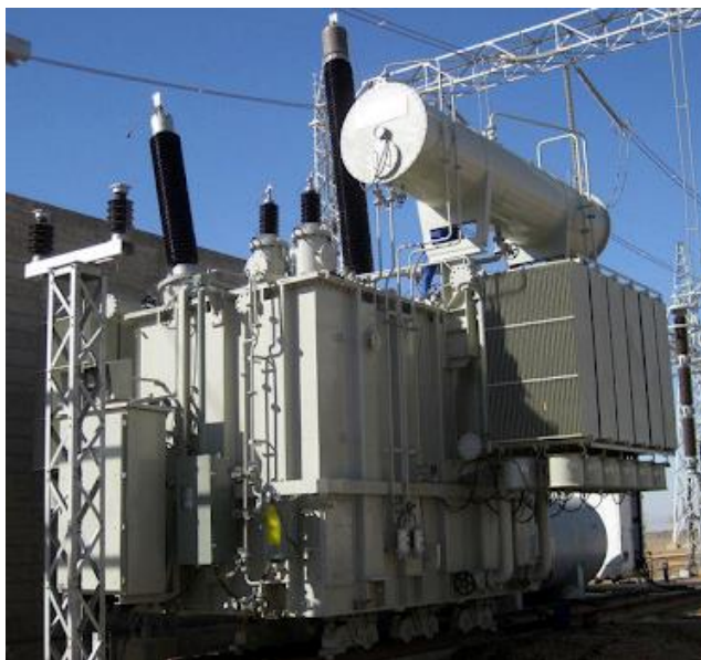
Gambar 2.10 Transformator Daya
