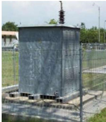
Gambar 2.10 Neutral Grounding Resistor
