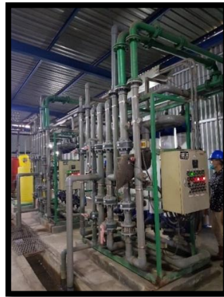
Gambar 2. 7 Demineralization Plant (Sumber: Dokumentasi Pribadi)
