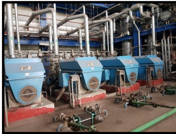
Gambar 2. 26 Feed Water Pump (Sumber: Dokumentasi Pribadi)
