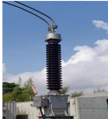
Gambar 2.4 Potential Transformer 7
