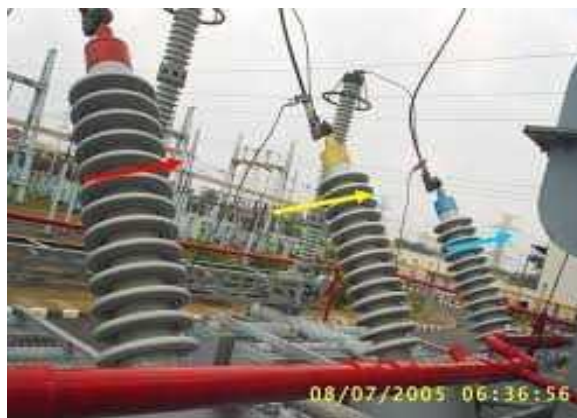
Gambar 2.13 Bushing Transformator
