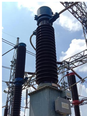
Gambar 2.3 Current Transformer
