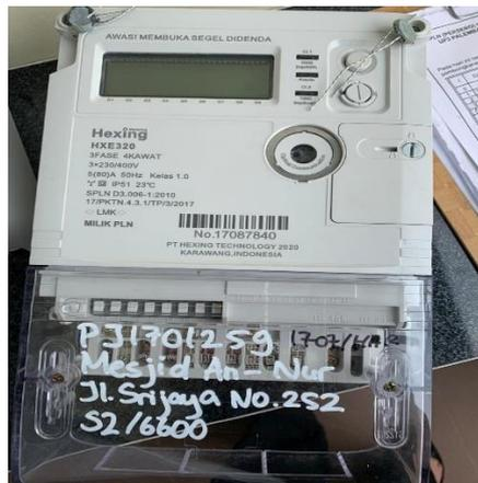
Gambar 2.13 Kwh Meter 3 Phase
