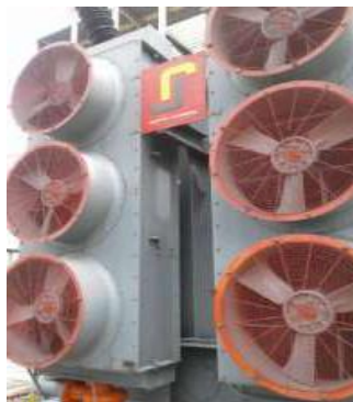
Gambar 2.12 Pendingin Transformator
