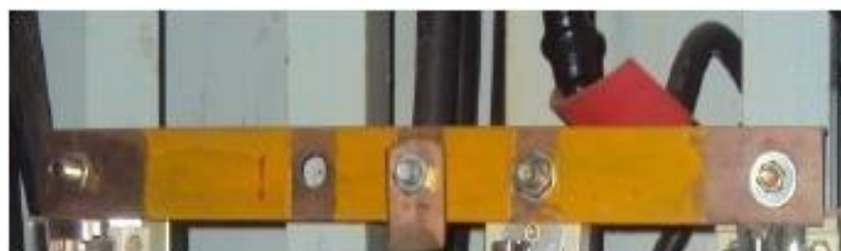
Gambar 2.4.2 Terminal Pbumian
