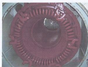
Gambar 2.3 Stator Generator (6)
