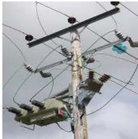
Gambar 2.11 Load Break Switch (LBS)
