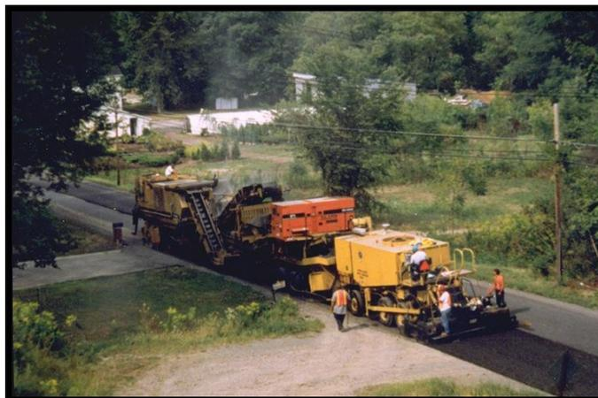
Gambar 2.10 *Cold in-place Recycling*
