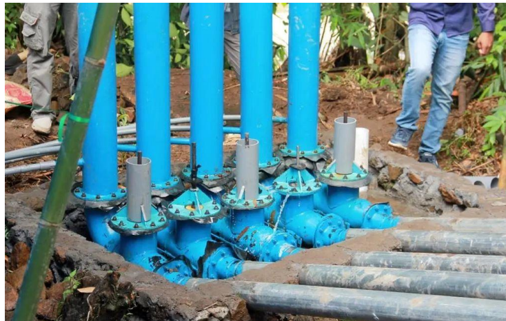
Gambar 2.1 Hydraulic Ram Pump (Sumber: www.Bengkuluinteraktif.com , 2022)
