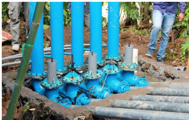
Gambar 2.1 Hydraulic Ram Pump (sumber: Alfridho, 2022)
