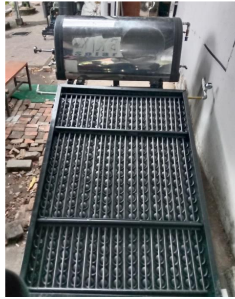
Gambar 18. Solar Water Heater Tampak Atas
