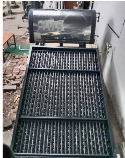
Gambar 5.18. Solar Water Heater Tampak Atas
