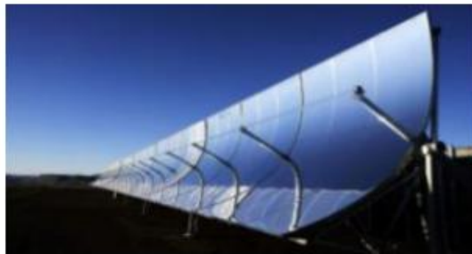
Gambar 2.3 Concentrating Collector Sumber : Infostudikimia.com
