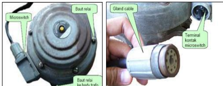
Gambar 2.18 Rele Sudden Pressure 30
