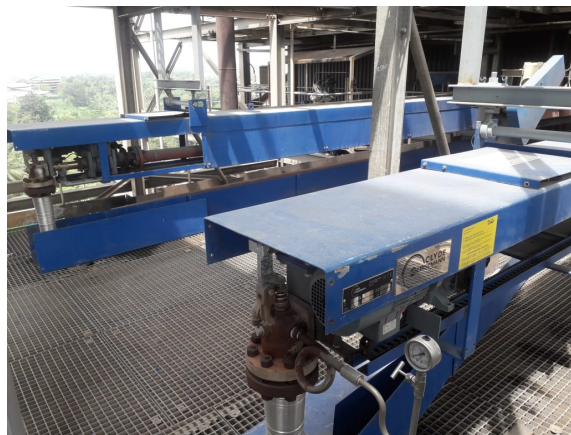
Gambar 2.11 Long retractable sootblower
