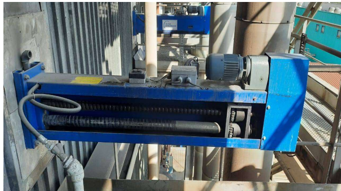
Gambar 2.13 Half Retractable Sootblower.
