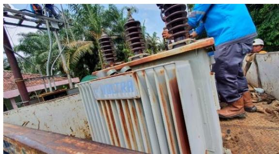
Gambar 2. 10 Transformator Distribusi Tiga Fasa
