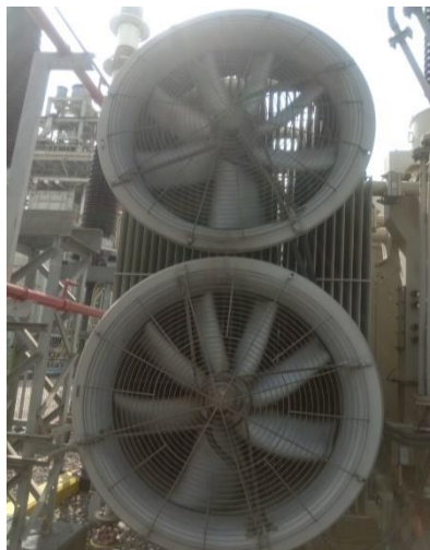
Gambar 2.11 Pendingin Transformator
