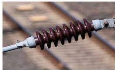
Gambar 2.6 Isolator Tarik Polimer dan Isolator Tarik Porselin
