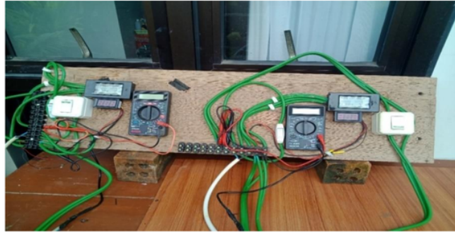
Figure 3. Circuit and installation of measuring tools
