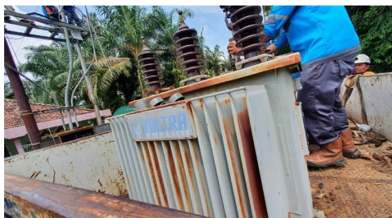
Gambar 2. 10 Transformator Distribusi 3 Fase
