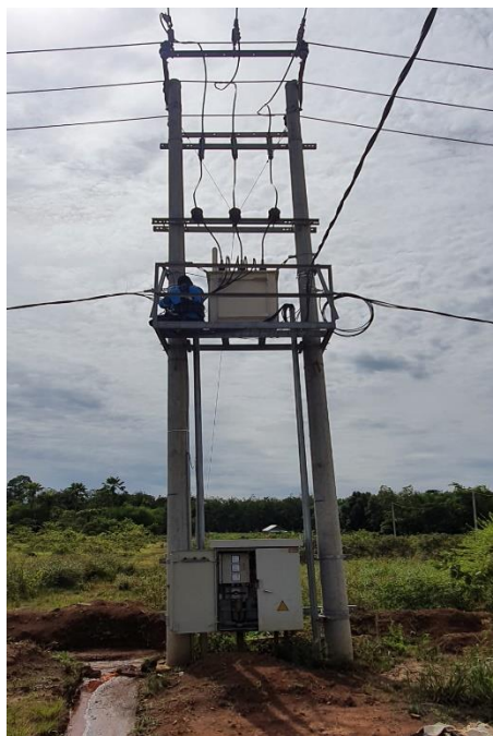
Gambar 2. 1 Gardu distribusi dan Single Line Diagram
