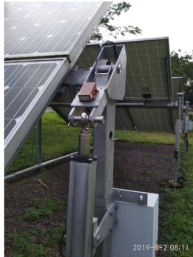
(b) Installed solar tracker and actuator in PV system
