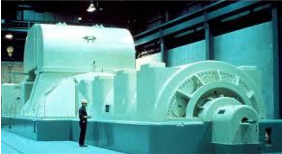
**Gambar 2.4** Generator Sinkron
