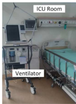
Fig. 10. Ventilator and monitors as the load for PV system considered in this study
