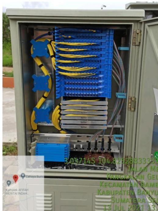
Gambar 2.6 *Fiber Distribution Terminal (FDT)* [7]
