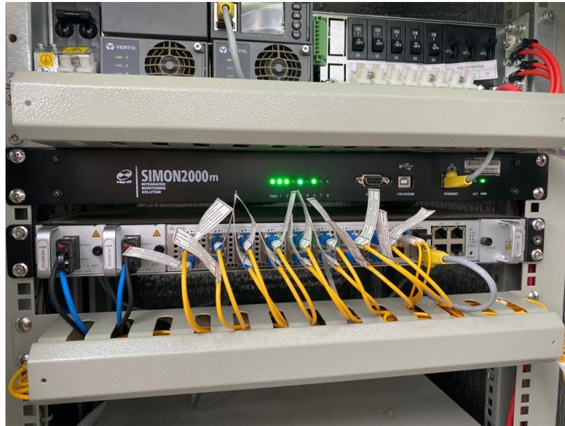
Gambar 2.5 *Optical Line Terminal (OLT)* [7]
