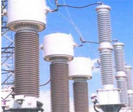
Gambar 2.5 Transformator arus
