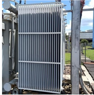
Gambar 2. 6 Pendingin transformator
