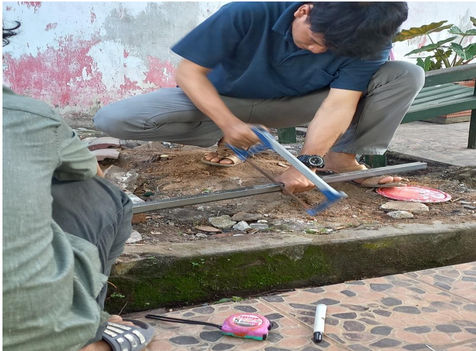
LAMPIRAN 2 Pematongan Rangka Tiang Weather Station
