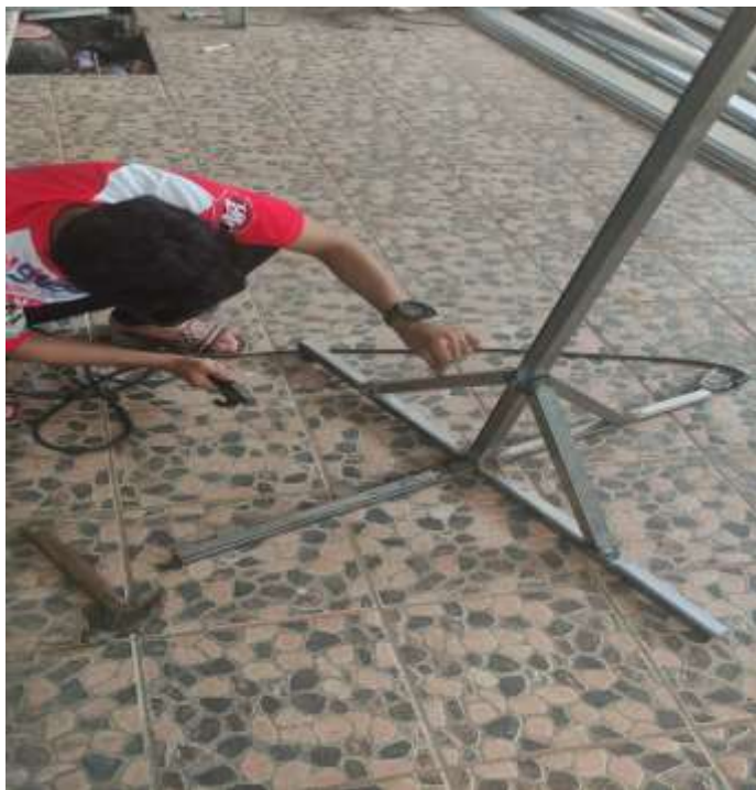
LAMPIRAN 3 Pengelasan Tiang Weather Station
