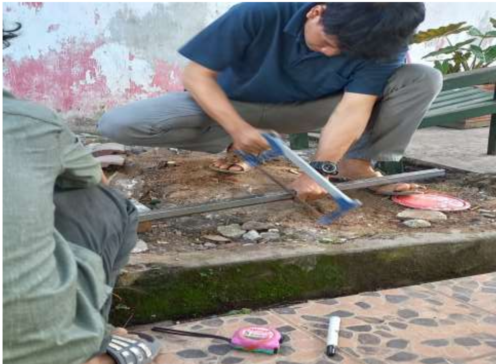
LAMPIRAN 2 Pemotongan Rangka Tiang Weather Station
