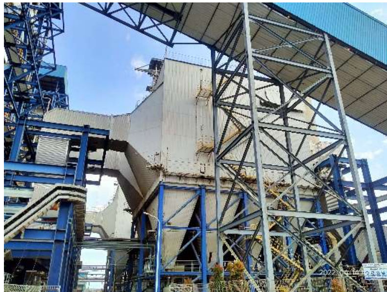
Gambar 2. 1 Electrostatic precipitator (ESP)
