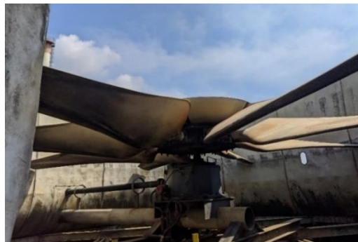
Gambar 2.15 Axial Fan di PLTGU Keramasan
