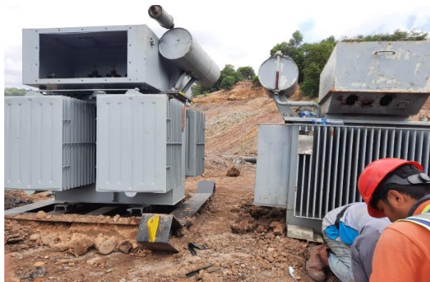
Gambar 2.1 Transformator Distribusi
