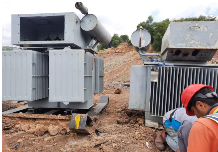
Gambar 2.16 Transformator Distribusi
