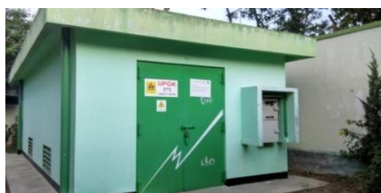
Gambar 2.3 Gardu Beton
