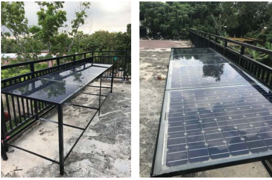
Figure 1. Mono Si PV Solar Panel Unit Installation
