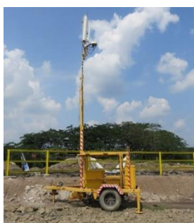
Figure 1. The mobile tower deployed in the open-pit mine.
